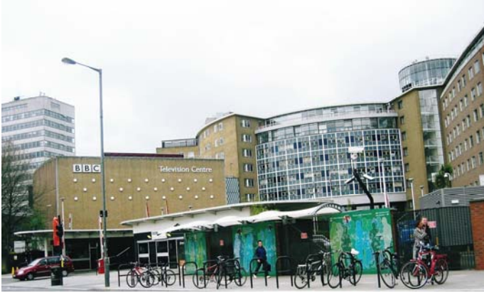
Appearance of the building
