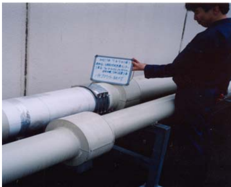
PT- 200DS on iron pipe of 200mm in diameter
