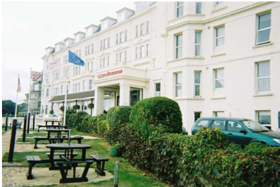
Appearance of the building
